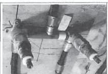
Cutaway behind the wall showing exposed shower spindle and spindle extension used to operate the shower. An investigation into the water leak is ongoing but has revealed loose spindle and/or spindle extensions
