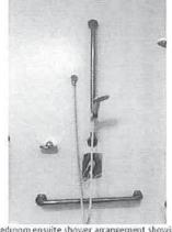
Bedroom ensuite shower arrangement showing mixer and in-wall box to operate the shower as the replacement for the spindle arrangement.
