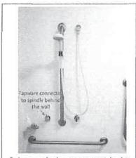
Bedroom ensuite shower arrangement showing tapware that is connected to spindles used to operate the shower.
