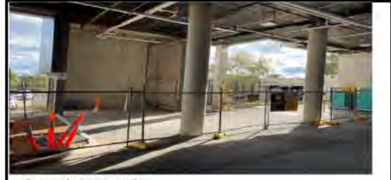
Fire Control Room Construction
